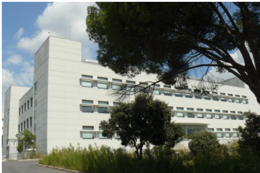
Fig.12: CBGP Building in Montegancedo Campus
